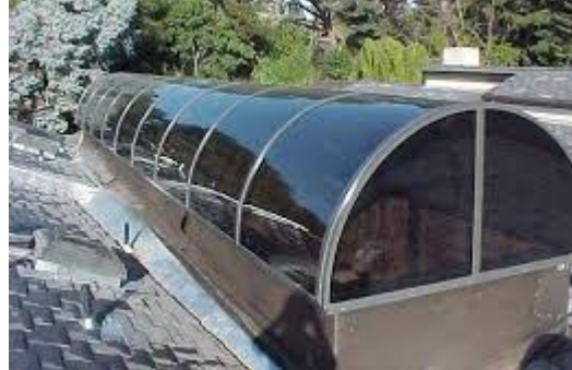
Figure B - Typical commercial barrel-vault skylight
