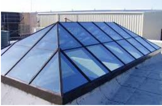
Figure A - Typical commercial hip-ridge skylight
