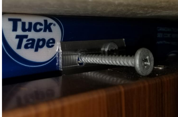
Installation Photo – Top installation clip
