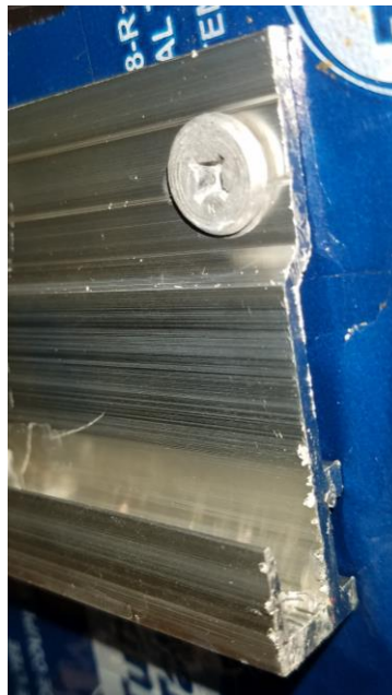
Installation Photo – Starter J-Track
